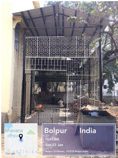
Newly constructed workshop (Ceramic & Glass)
